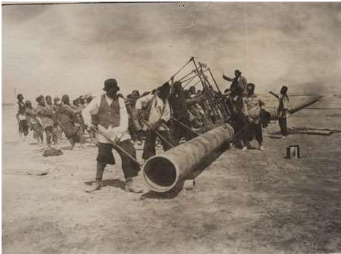
D'Arcy builds a desert pipeline to Abadan...
